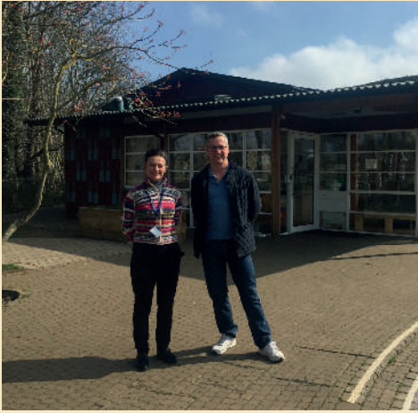
Driven by Cllr Bridget Smith, the Gamlingay Eco Hub is the country's most energy efficient community building, bringing together parish office, library, sport and social groups.
