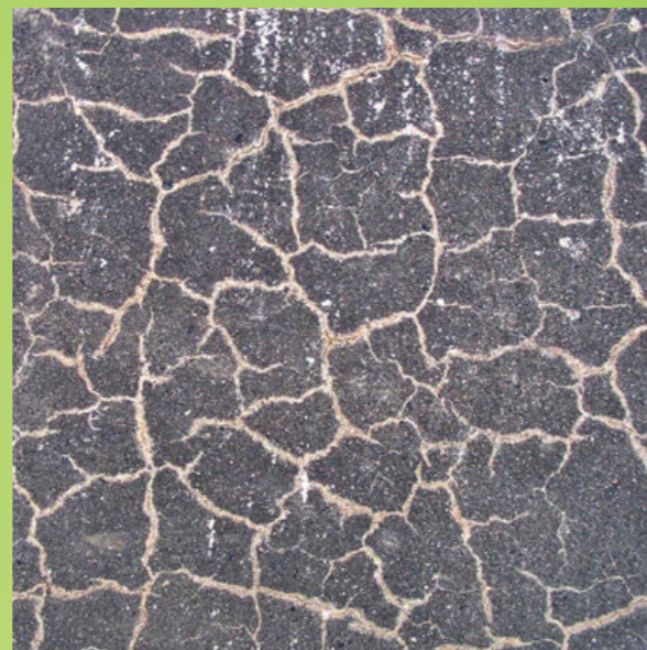
CRACKING
