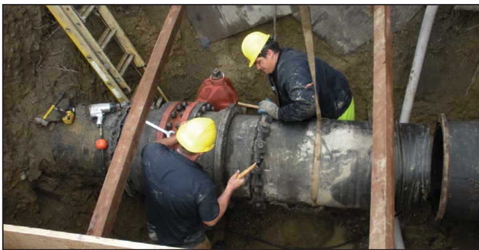
City of Kent Water Department installing 24" butterfly valve on incoming side of their water supply to the valley floor.
