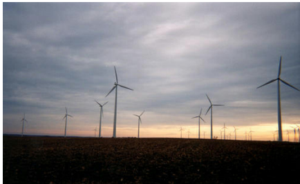
Top of Iowa Wind Project. Photo courtesy of NREL
