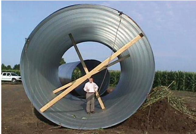
Steel tube which makes up a portion of the foundation of Carlton College's 1.65 MW wind turbine.
