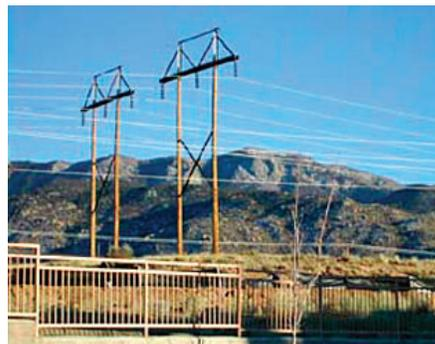
*230 kV transmission line. Notice the three wires or conductors hanging from each tower. Three or four wires generally will signify a three phase transmission line.*
