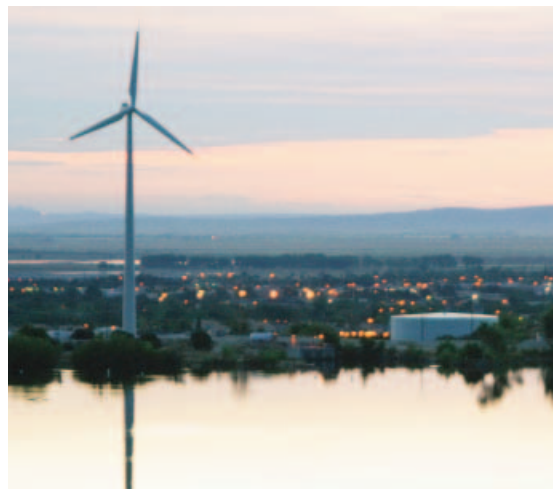
Palmdale Water District uses the power from this 950 kW turbine to provide electricity for the municipal water treatment plant 50 miles north of Los Angeles, California.
