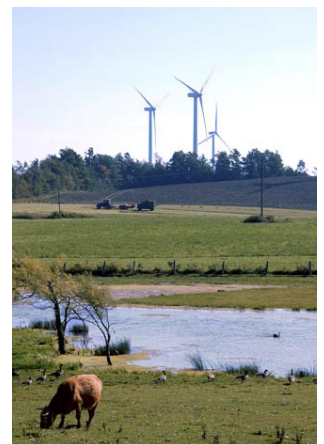
A New York State wind project.
