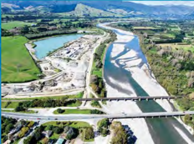
Peka Peka to Ōtaki Expressway - design management, environmental and stakeholder management, geotechnical design, stormwater design and ecology
