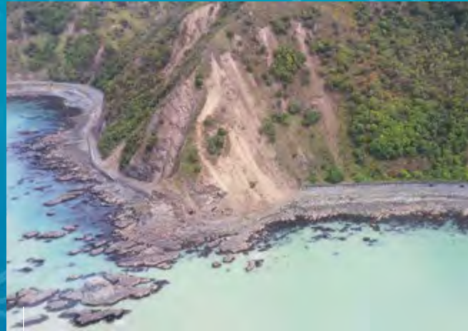
North Canterbury Transport Infrastructure Recovery (NCTIR) - environmental management, planning, approvals, ecology, coastal and geotechnical engineering and geology
