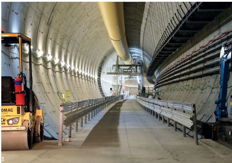
1 Waterview Connection Tunnel 12d is being backfilled as it progresses. 2 Waterview Connection Tunnel entry. 3 Western Ring Route.
