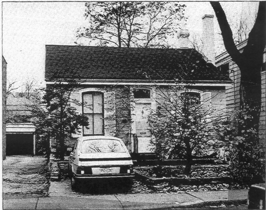
23 Boswell constructed in 1877 first resident: Joseph Nichols, carpenter.
