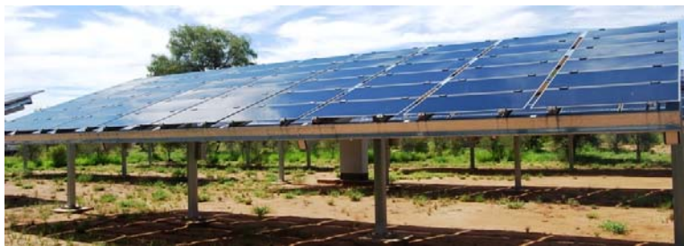
Figure 1: Calyxo CdTe thin film array
