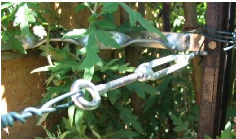
Turnbuckle hook fastened to a secure wire loop on bracket where bolt occupies hole is star picket
