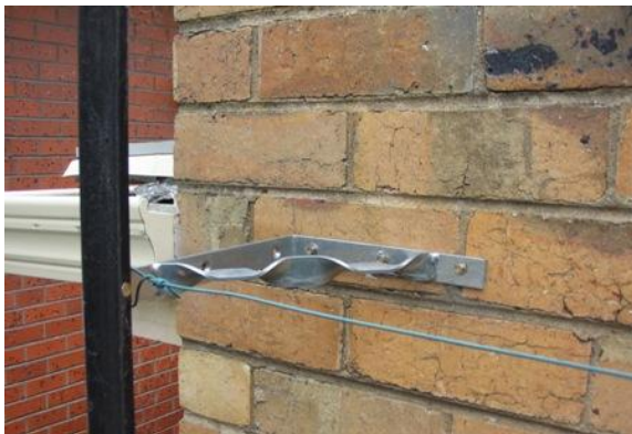
Braced bracket for extra strength, mounted horizontally and facing inwards for maximum strength. One bolt fastens the star picket to the bracket. Since the bolt occupies the hole on the star picket, the wire is fastened around the end of the bracket.
