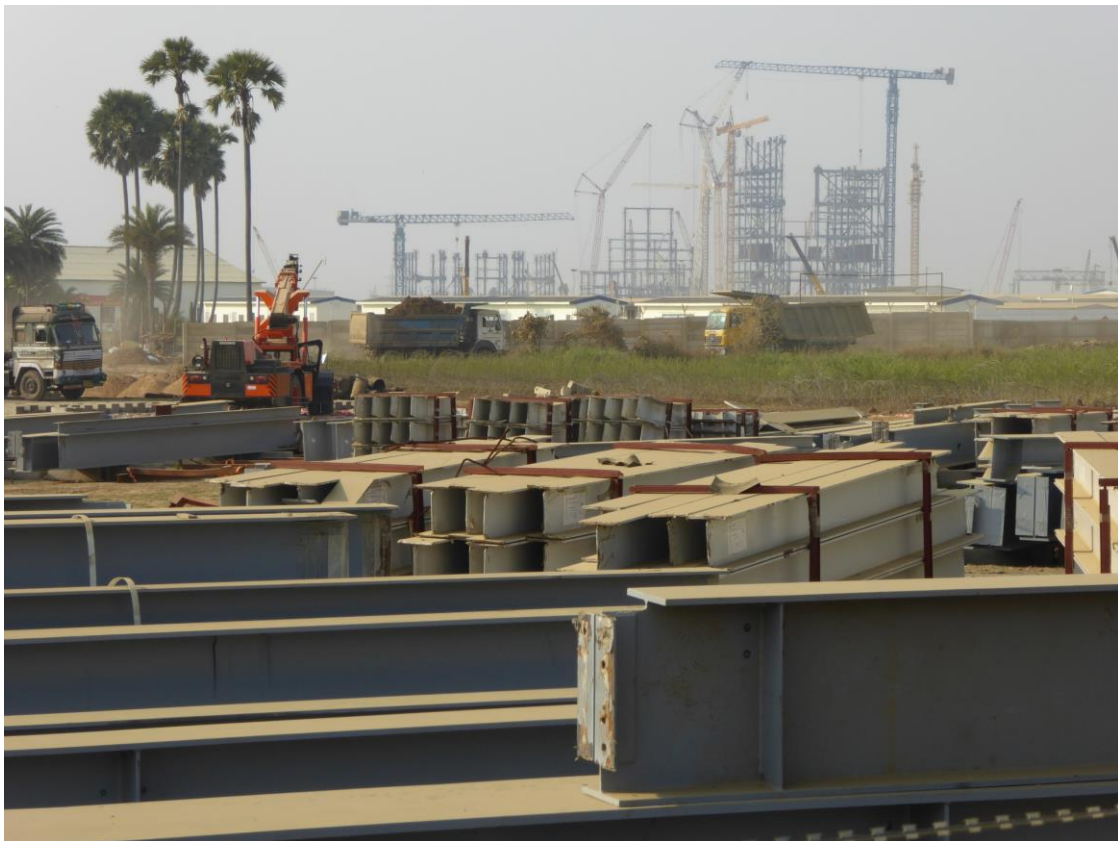
Construction of Adani’s Godda power station proceeds on lands acquired from indigenous farmers near Godda. Photo by Geoff Law, February 2020
