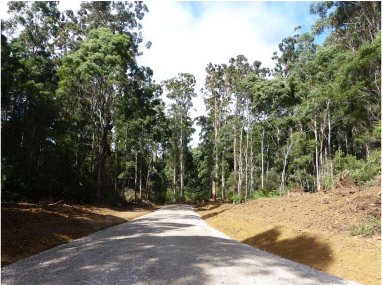
Below: Same Road on 8/2/2017, showing continuation of roadworks (gravel laid).
