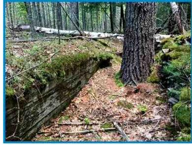
**Wagon Road Engineering:** Quarry workers went to great effort to engineer roadbeds suitable for heavy wagon traffic. A discerning eye will notice short and long road sections filled, graded, or entirely constructed with quarry rubble (to 250<sup>+</sup> feet), ramps crossing low wetlands and grading to quarry exposures (right), notched hillslopes, and loops constructed to connect quarries and direct wagon flow.
