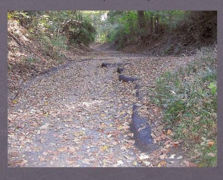
The crushed stone is deposited elsewhere on the trail to form bicyclist "sand traps"
