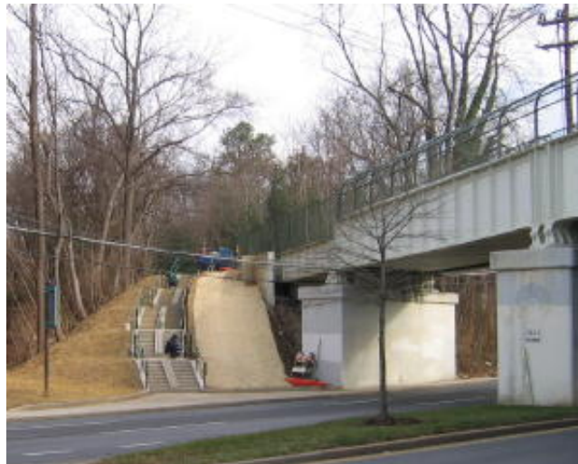
The new access staircase on the north side of Bradley Blvd.
