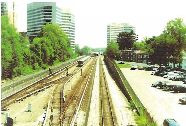
Figure 55: Looking south from Spring Street Bridge
