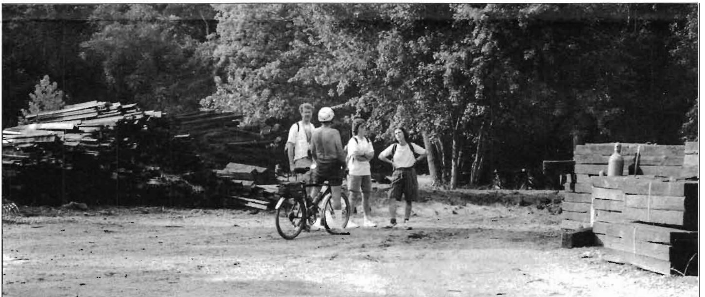
Rails and ties are stockpiled near Fletcher's Boat House.
