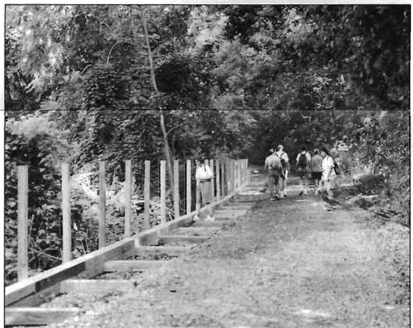
Viewing progress in the District portion of the corridor.
