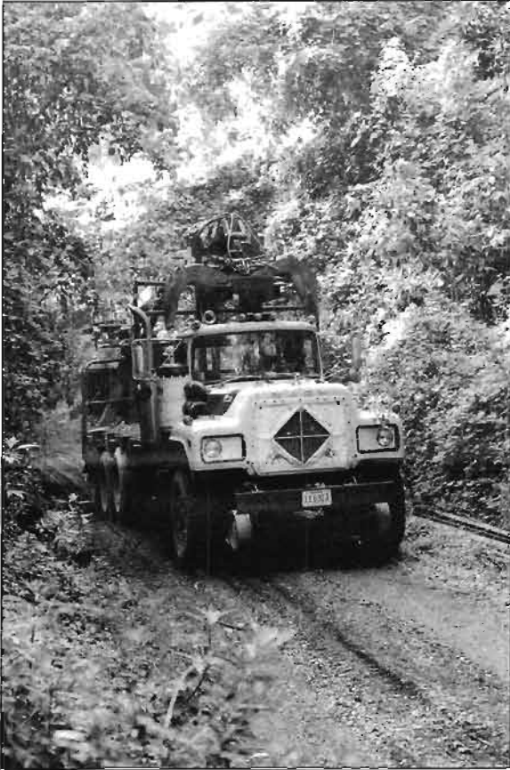
Heavy equipment was brought in by contractors to remove rails.
