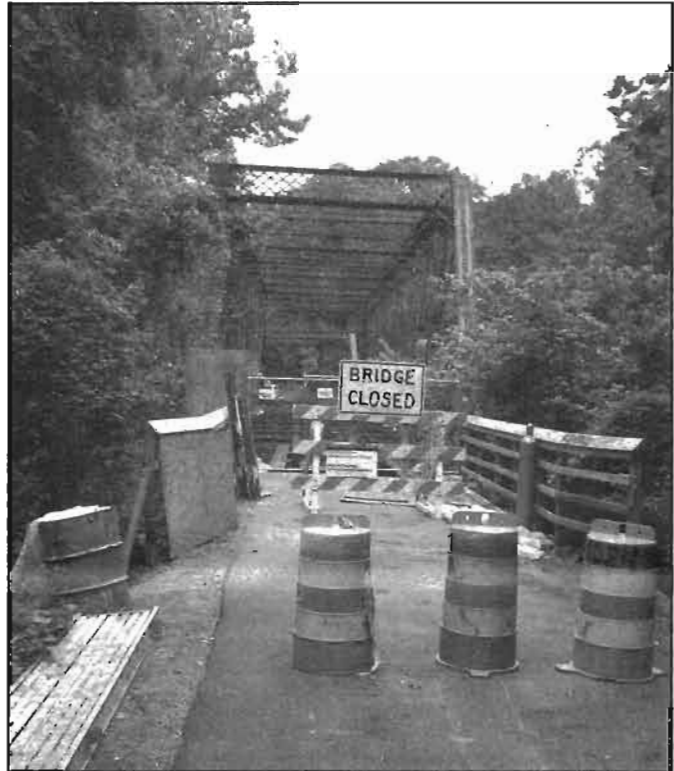
Construction began on the Arizona Avenue Trestle in May but no visible signs of progress were displayed in July. Photo: Chris Brown
