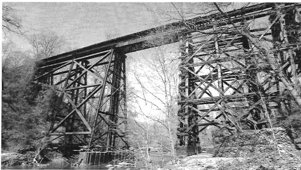
A March 1996 view of the trestle from the south emphasizing its impressive size and showing the 1972 steel construction on the left. Photo by G. Frederick Stork
