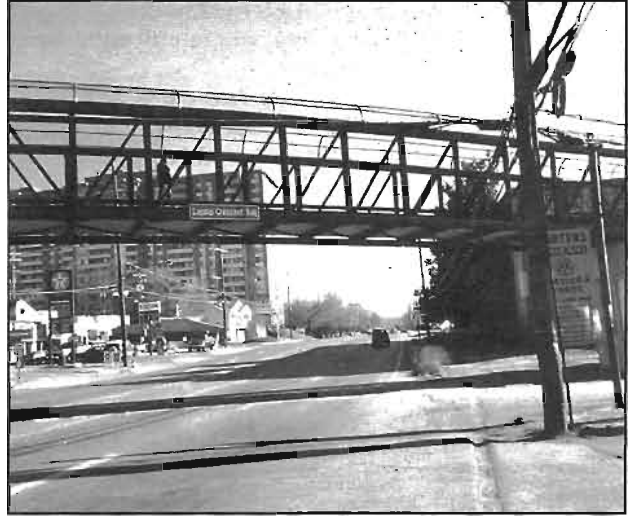
River Road Bridge
