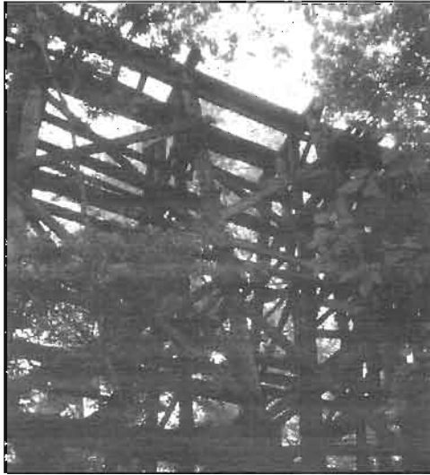
The trestle's wood support beams and columns on its east side (left) and the steel support on its west end (right).
