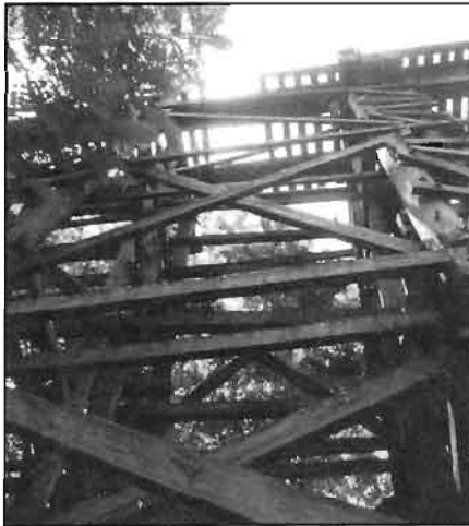
The trestle wood substructure will remain for historic and architectural purposes.
