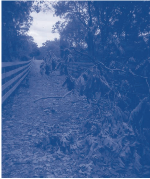
The trail's approach to the Rock Creek Trestle, after a summer's storm.
