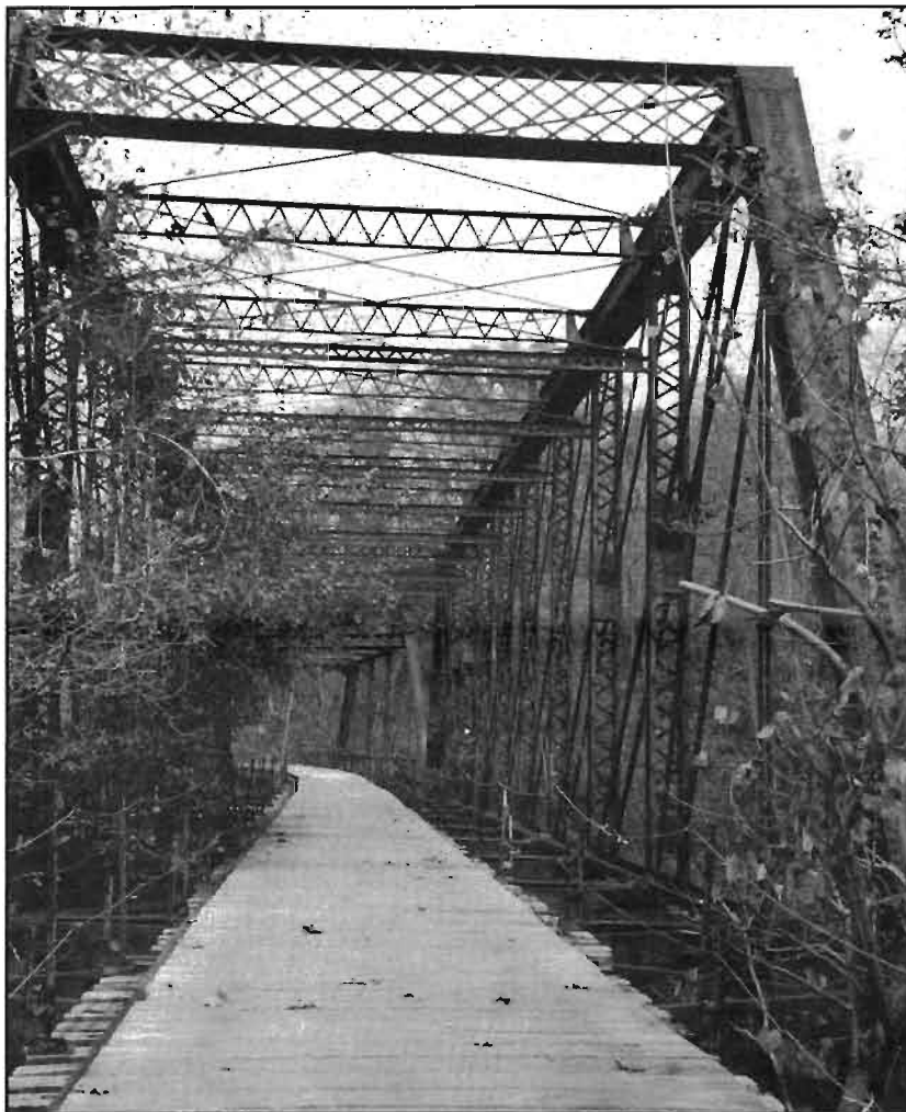
The curved Arizona Ave. trestle posed challenges for engineers trying to fit the Capital Crescent into the palisade shelf in the 1800s. The paved portion will be wider than it appears above when completed this fall. Photo by Tom Barrett.
