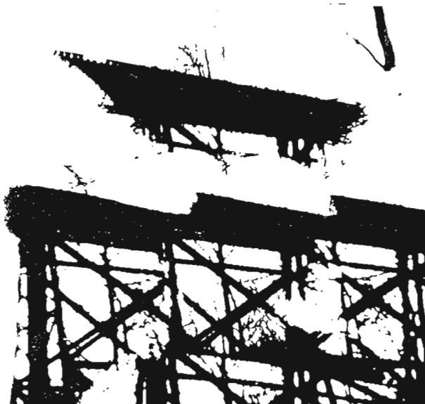
This picture taken with a quintuple filter shows the artistic possibilities of an interesting subject like the trestle. Photo: G. Frederick Stork
