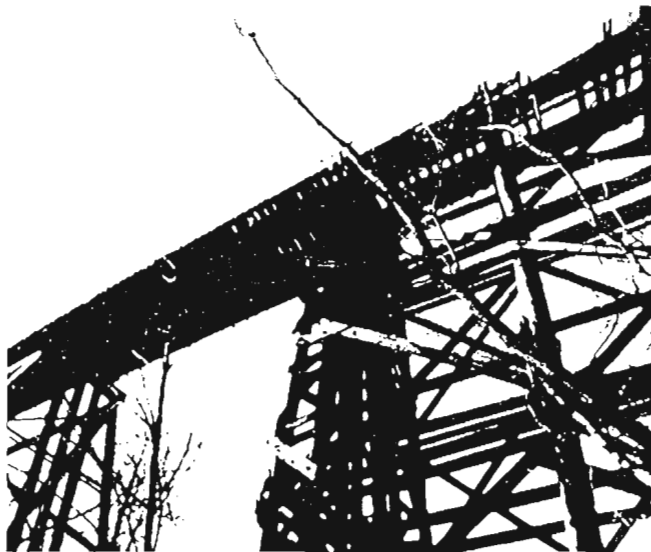
The one-track trestle bridge over Rock Creek in Chevy Chase as it looks today. The picture was taken from the bicycle path on the east side of the creek with the camera facing northwest. Photo: G. Frederick Stork
