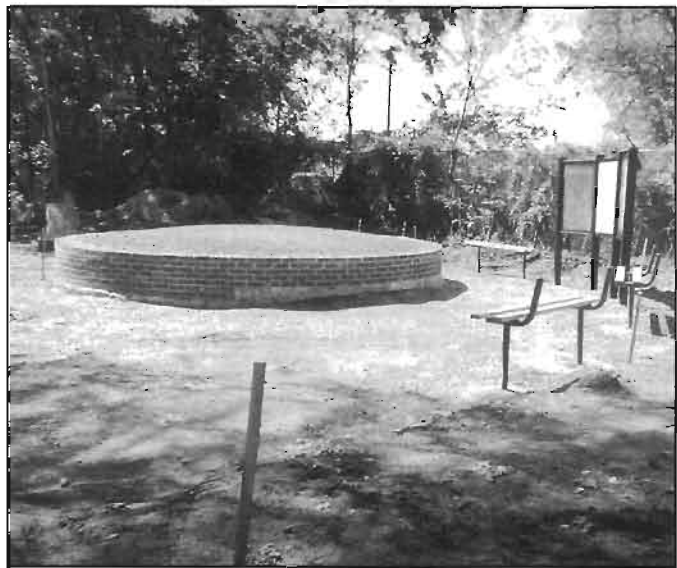
The Bethesda rest stop during the construction phase last fall.
