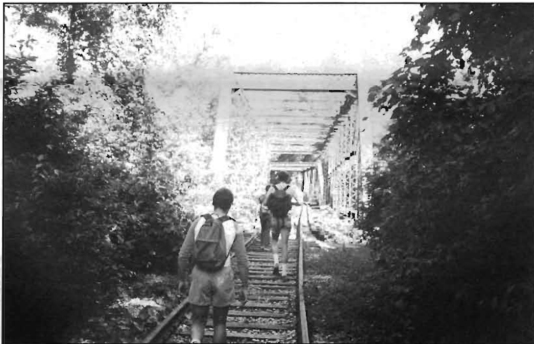
The Arizona Avenue trestle
