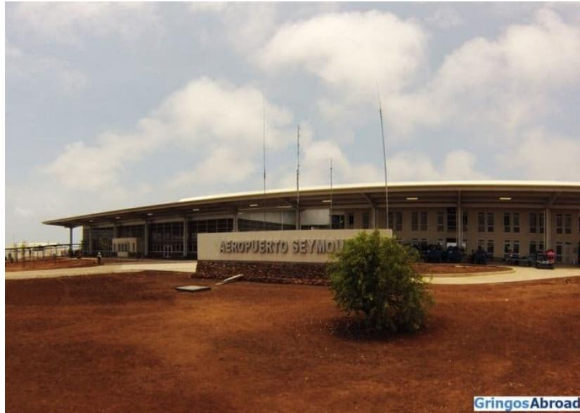
A lot of recycled material (80%) was used in the construction including steel tubes (from oil drilling in the Amazon) and material from the former airport. It operates on solar and wind power. There are small souvenir shops and a restaurant at the airport.
