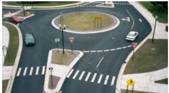
A roundabout is a raised circular island in a major intersection with deflector islands to slow approaching vehicles and provide crossing area.
