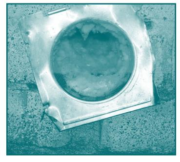
Build up of lint in dryer vents can cause fires and excessive heat in dryers
