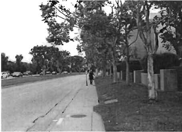
The narrow sidewalk on Olympic Boulevard brings traffic uncomfortably close to pedestrians.
