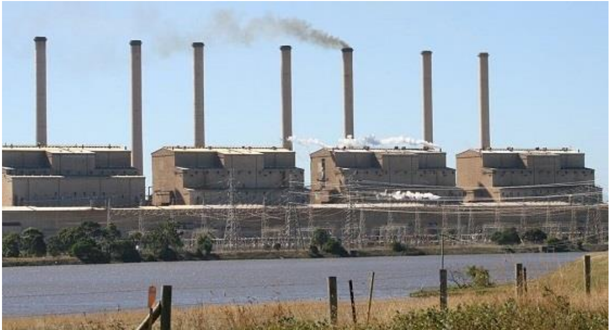
Hazelwood power station. Photo by Mriya, Wikipedia.
