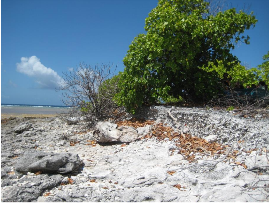
Erosion (Wenete village)
