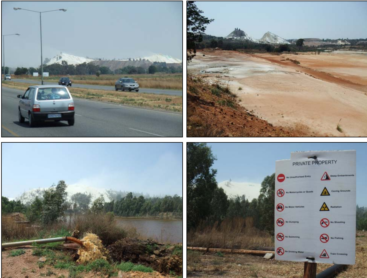
Figure 6: Radioactive gold tailings in the West Rand, Johannesburg, South Africa, showing major dust, radiation, safety and acid mine drainage problems (October 2010; all photos author).
