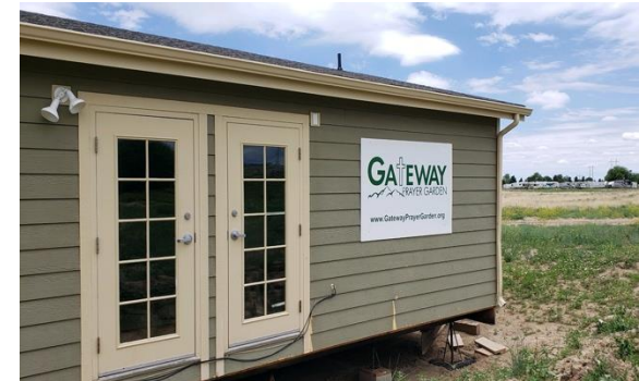
New On-Site Security-Construction Office!
