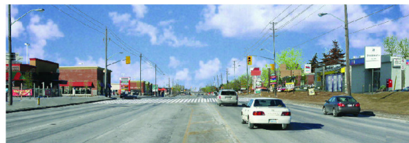
Before intensification and revitalization of an arterial road.
