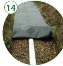
14 Soakaways, infiltration trenches & chambers
