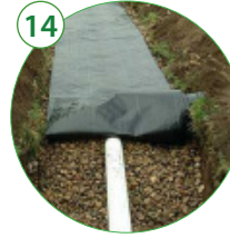
14 Soakaways, infiltration trenches & chambers
