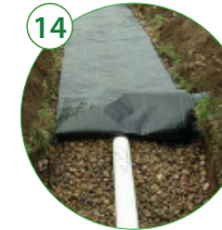
14 Soakaways, infiltration trenches & chambers
