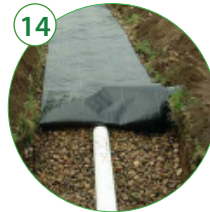
Soakaways, infiltration trenches & chambers
