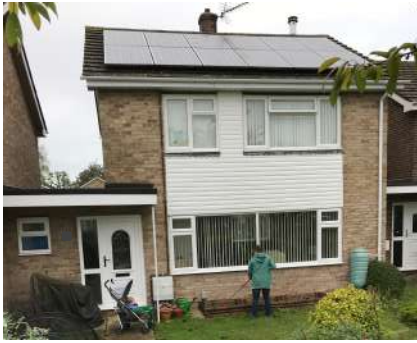
Clean energy: solar panels on a house in Witney North
