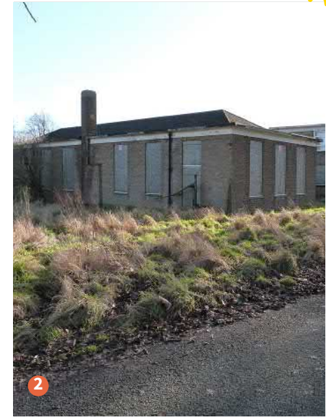
Opening up existing buildings
