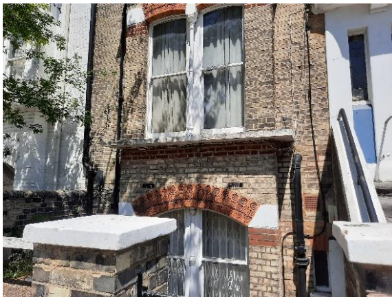
Decorative window railing is missing on the left-hand side
