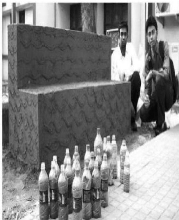
A bench built using plastic bottles filled with sand at Taramani | MARTIN LOUIS
