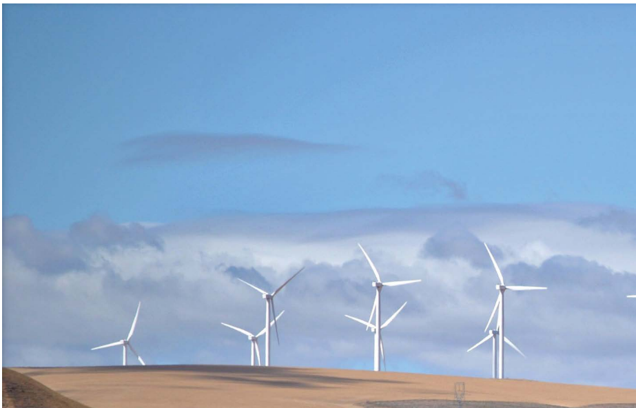
Shepherds Flat Wind Farm, Oregon, USA, seen from the Empire Builder train route. Credit: Steve Wilson, cc-by-2.0
