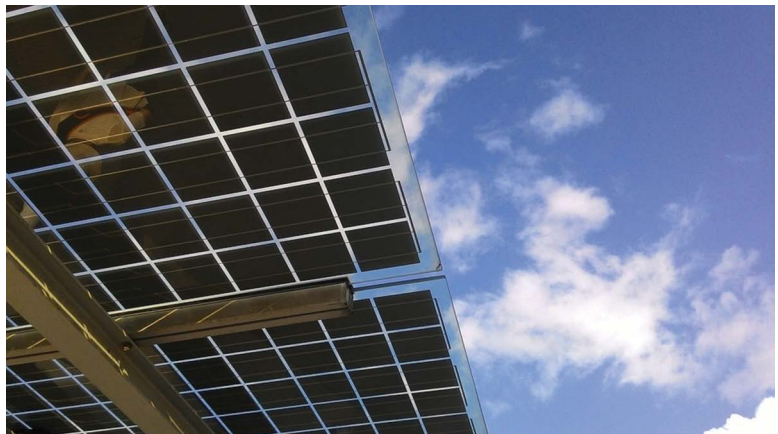
Double glass photovoltaic solar modules, installed in a support structure. Credit: Unsplash, cc0 1.0
