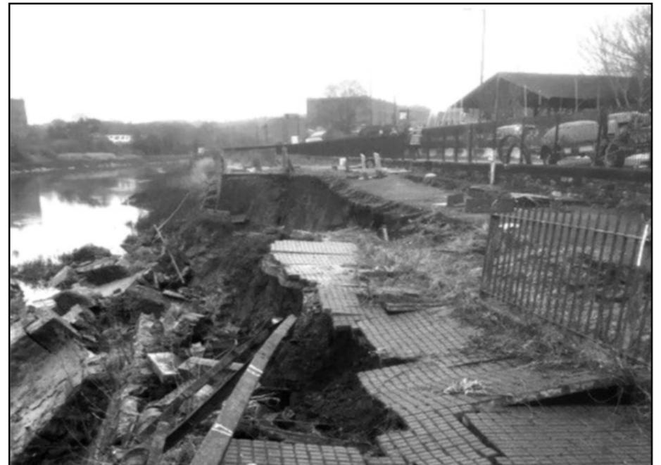
↑ The collapsed section of riverbank has taken the chocolate Path and railway track with it. It has been unstable for 3 years...
