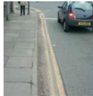
Grade C Widespread distribution of detritus with minor accumulations
