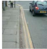
Grade C Widespread distribution of debris with minor accumulations
