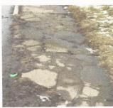
Level 1: Poor condition. Cracks and large vertical displacement.
