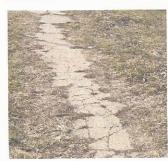
Level 0: Totally deteriorated or nonexistent. Serious surface defects.
