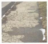
Level 2: Below average to average condition. Wide sidewalk cracks and small vertical displacement.
