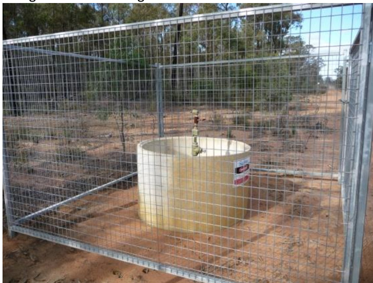
High point vent in Narrabri Gas Project flow line
